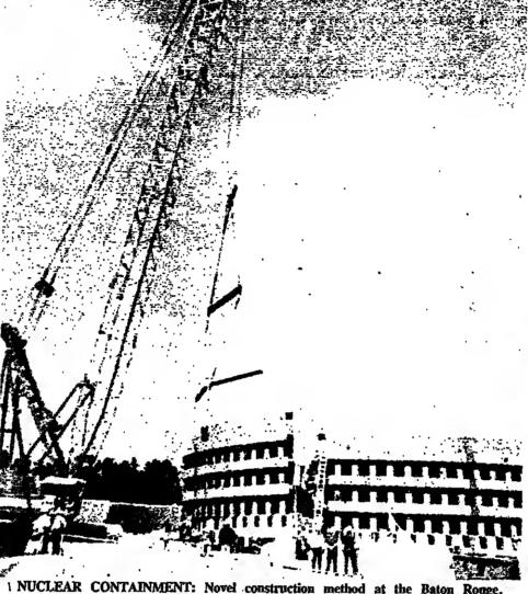
NUCLEAR CONTAINMENT: Novel construction method at the Baton Ronge, Louisiana nuclear power plant features the use of huge prefabricated containment sections weighing 90 tons. Each section is pre-plumbed and can be installed in a record amount of time.
